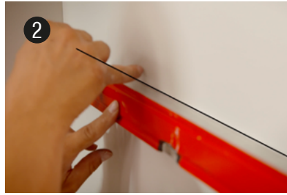
2 Mark out | Mark out the lines with a spirit level.
