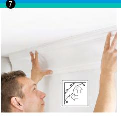
**Push firmly** I Ensure that you apply the marked edge to the ceiling. Put the crown molding into place, checking that it is horizontal and symmetrical to the wall and ceiling. When you are confident the molding is positioned correctly, firmly press it to the wall and ceiling across the entire length.
