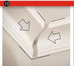
**Push** both moldings firmly and securely together. Excess adhesive should seap through the joint.
