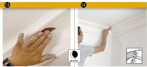
**Prepare for paint** I All Orac Decor® moldings are pre-primed in white, but still need to be painted over with a suitable paint. For good adhesion, lightly rub the length of the moldings with a 320 gram sandpaper.
