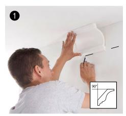
**Mark out** I Mark the bottom of the crown molding on the wall. Make sure the molding is positioned correctly at 90°.
