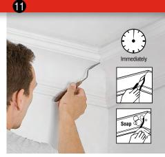
Clean | Clean excess adhesive with a painter's knife and soapy water within 10min after application.
