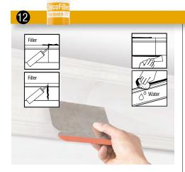
**Use DecoFiller to smooth out all visible joints** I If there are minor irregularities on your molding and/or wall joints these can be filled with our FL300. You might find it easier to do this 24 hours after the initial installation.
